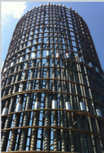
SimGrip Standard and Positional parallel threaded couplers in columns.
