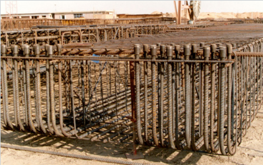
Linxion couplers in diaphragm wall.
