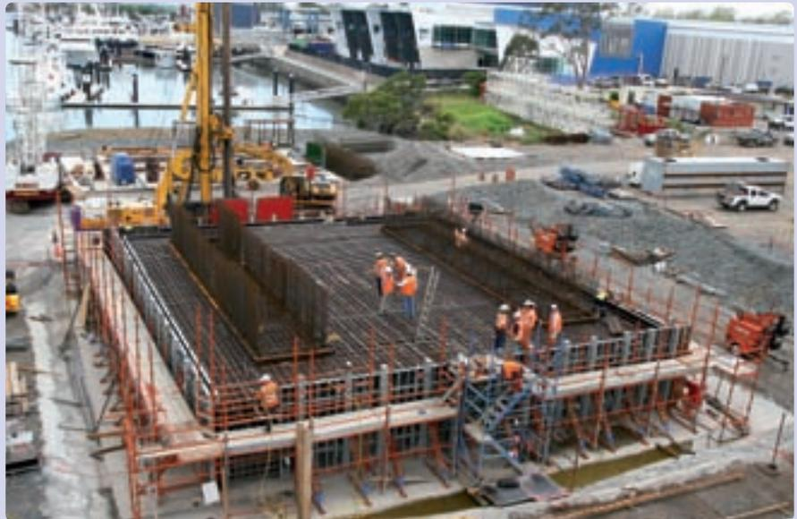
**Figure 1** Selective use of stainless reinforcement on the pile cap of the 300 year life Gateway Bridge, Australia, specified by Aecom using predictive modelling. Courtesy of Outokumpu
